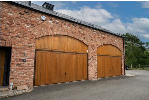
With an up and over remote control electric garage door, power and light.
